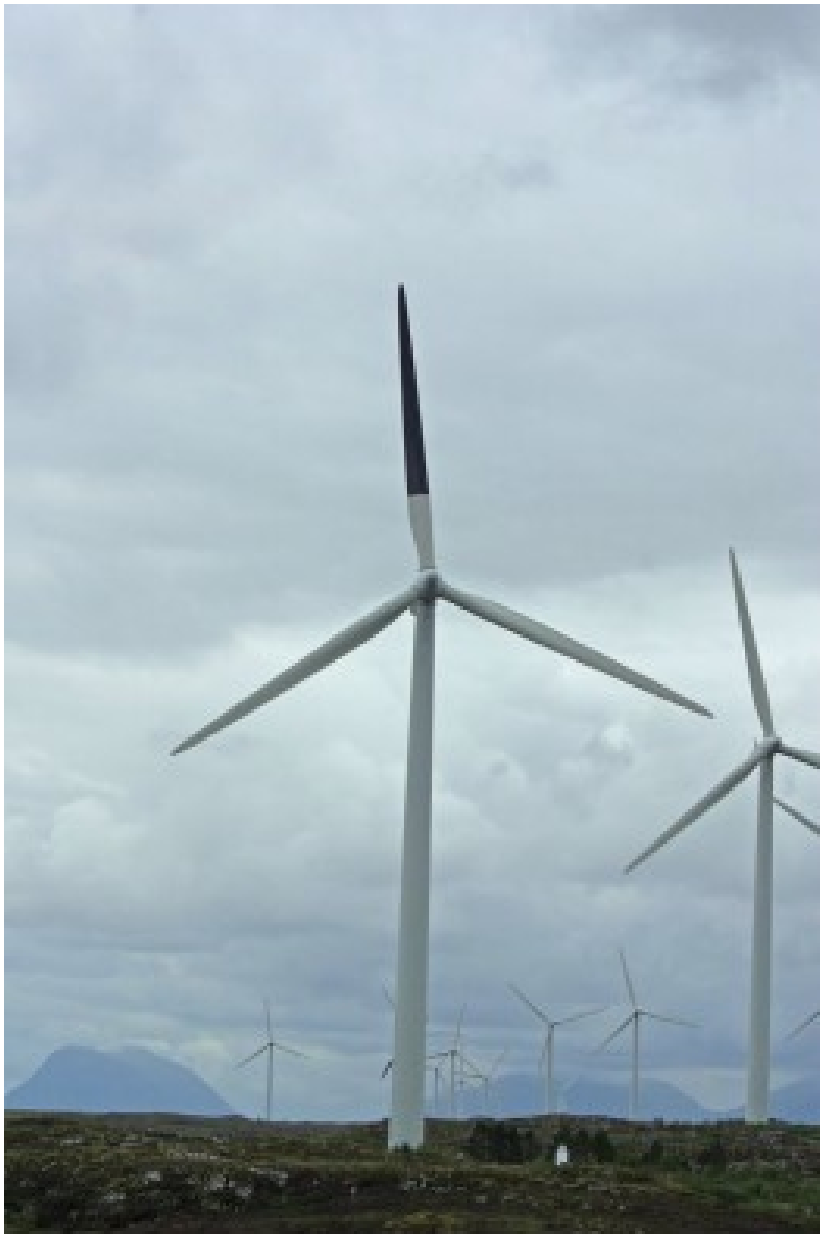
Foto: Wind turbine in the Smøla wind-power plant with painted rotor blade
